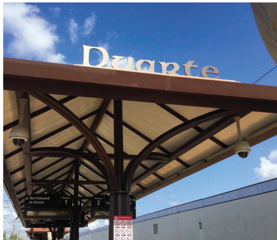
Duarte Metro Gold Line Station, located just south of the Specific Plan area
