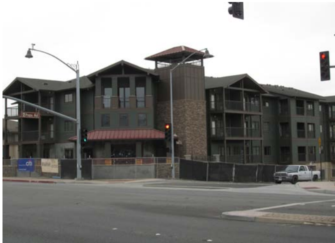
Phase II of Andres Duarte Terrace is currently under construction
