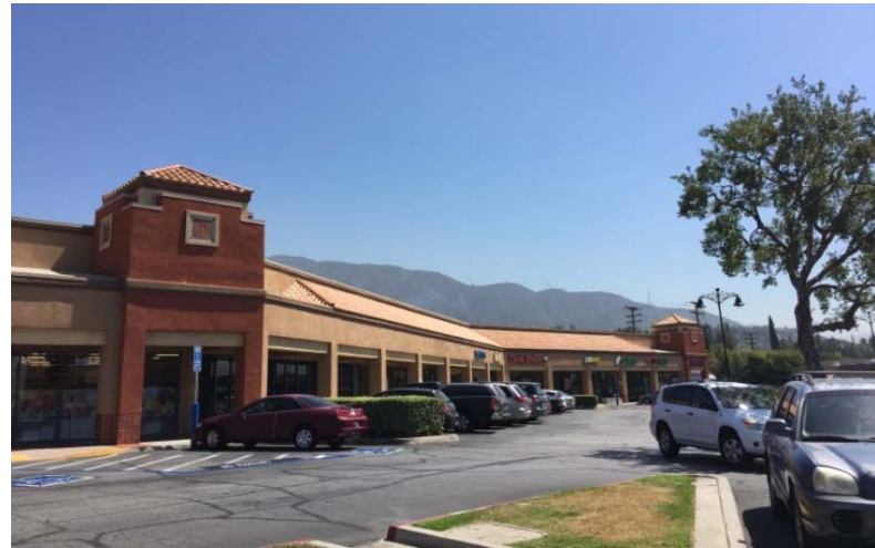
The Ralph's Center is newer and higher quality than other strip commercial
